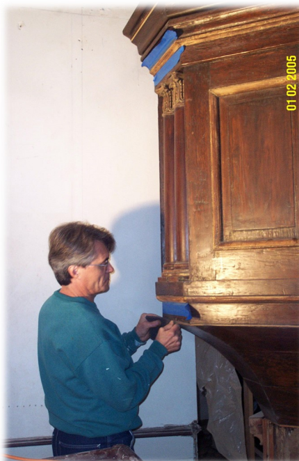
Pulpit repair, including fixing termite damage to the base and adding bolts to affix the top to the wall.
