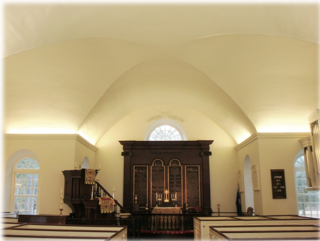
Barrel-vaulted ceiling above the crossing of the aisles.
