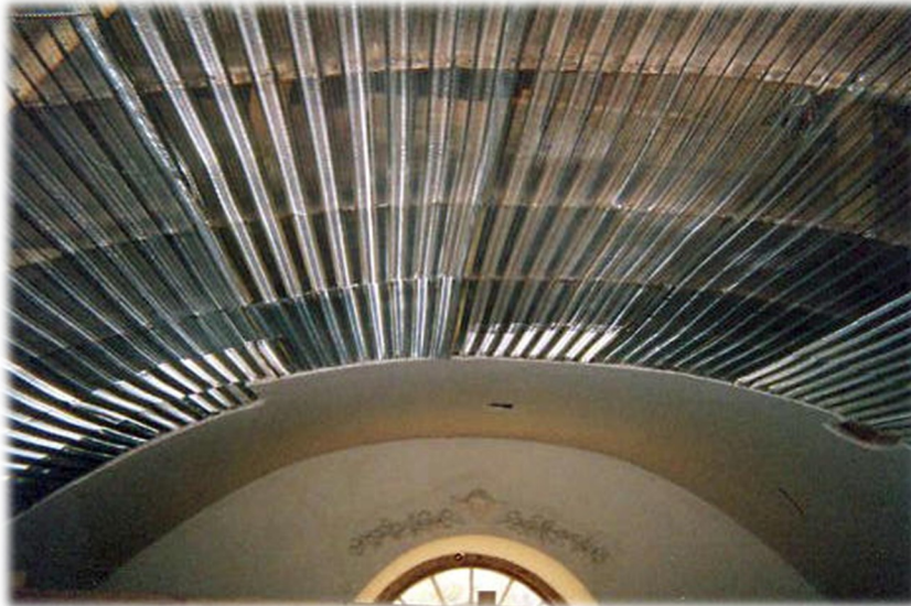
New steel lath ready for replastering.
