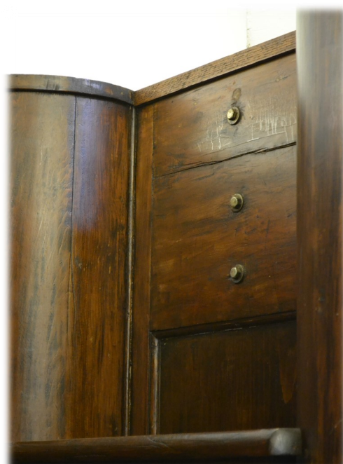
Pulpit repair, including fixing termite damage to the base and adding bolts to affix the top to the wall.
