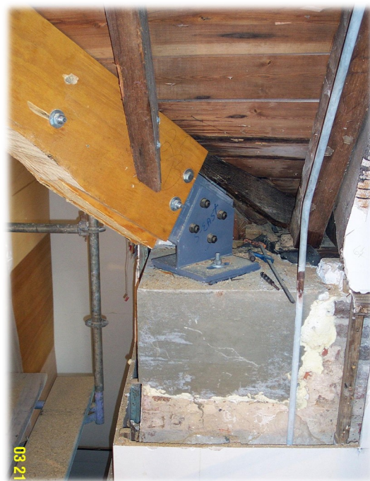
New roof truss base.
