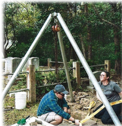
Grave of Mary C. Roach, students using a crane to reset the base.
