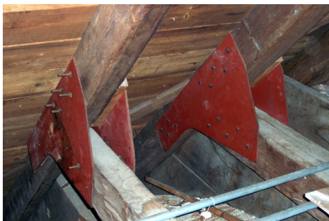
Repairs to the roof rafters: top and left, during the 2004–5 restoration; right, addition of steel gusset plates in 1960; courtesy of Richard Marks Restorations and Old St. Andrew's
