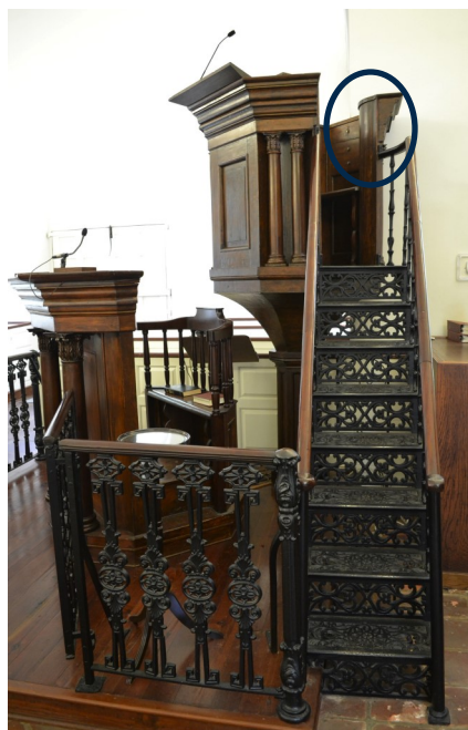
Bolting the pulpit to the wall: circled (top) and detail (left)
