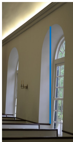
Colonial-style compass-headed window (top) and marked deflection when viewed at the crossing of the aisles (bottom)
