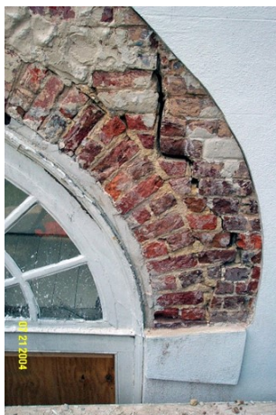
Stucco walls (left) and brick under stucco during 2004 repairs on the west wall (right), courtesy of Richard Marks Restorations and Old St. Andrew's
