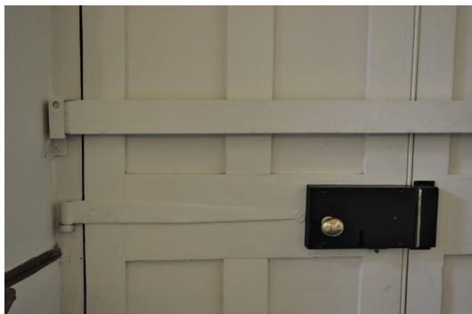
Church doors: north end (left), west end exterior (center), south end (right), and close-up of hardware and locking bar on north door (bottom)
