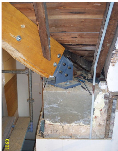
Repairs to the roof rafters: top and left, during the 2004–5 restoration; right, addition of steel gusset plates in 1960; courtesy of Richard Marks Restorations and Old St. Andrew's
